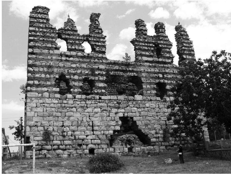
Fig. 3. Palace of Nymphaion, western façade.
